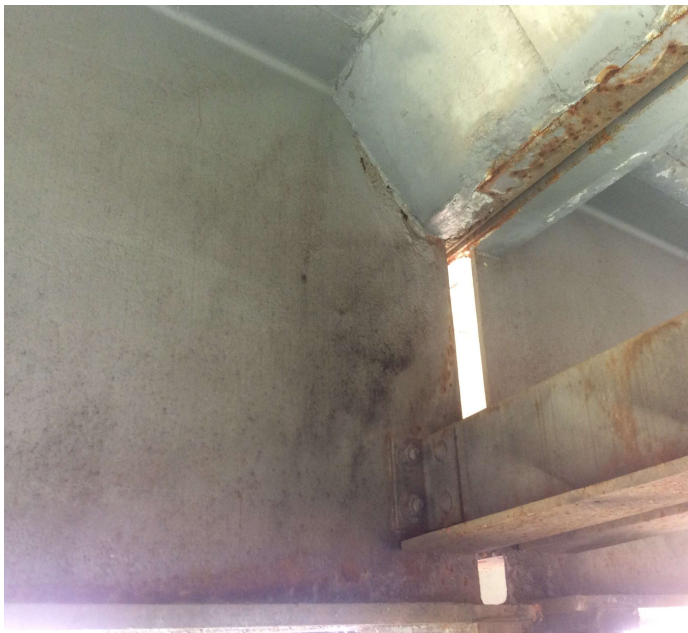
PHOTO 1 Description Painted over section loss
