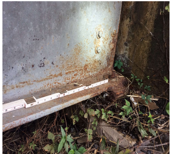
PHOTO 2 Description Span 4 girder 5, pitting up to 3/16" in web and bottom flange
