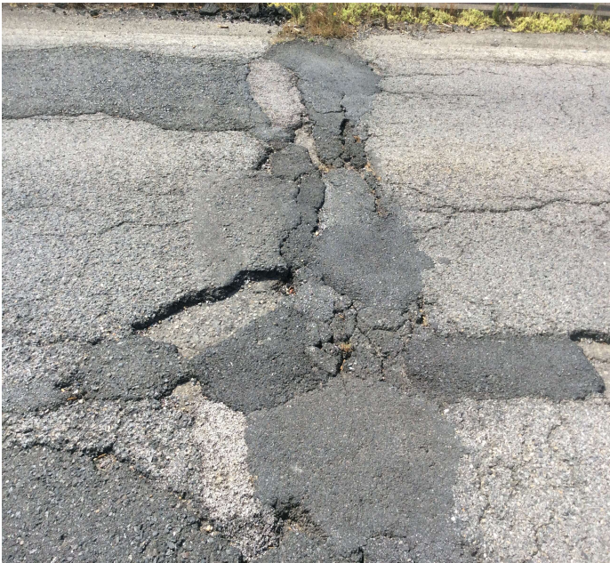
PHOTO 1 Description Asphalt overlay has large spalls and unsealed cracks
