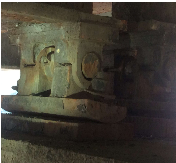
PHOTO 1 Description Span 2 at bent 2 bearings under girders 3,4 and 5 have a 1/8 inch gap around pins
